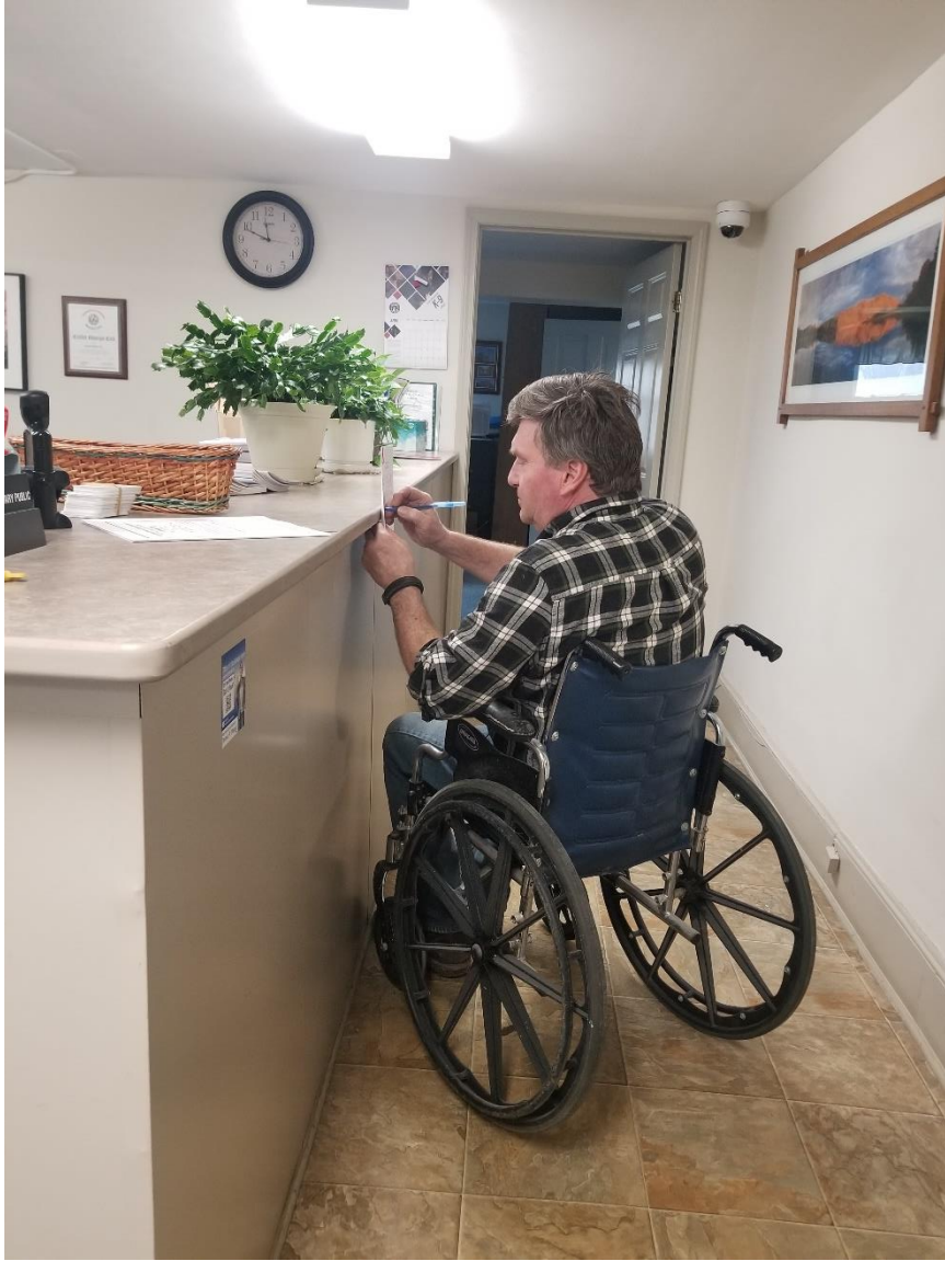
Main service counter is not ADA compliant
